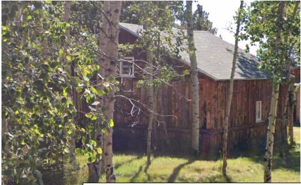
Figure 7: Detached Garage viewed from W. Kansas Alley in 2024
