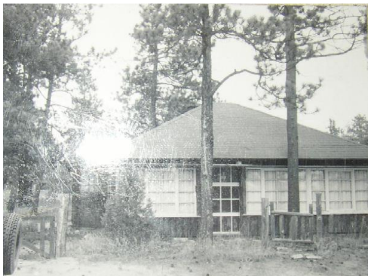
Figure 1: Griffith Cabin South Elevation – Circa 1965
