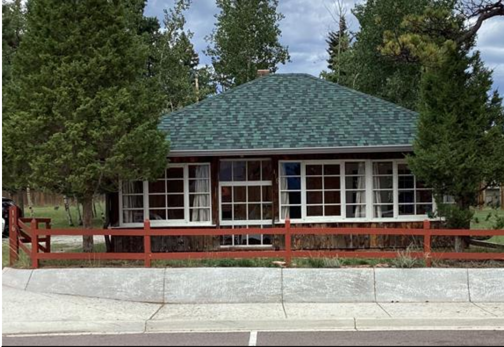
Figure 3: Griffith Cabin South Elevation 2026 – This elevation is an enclosed porch with multi-lite casement windows with fixed side Lites. A door opening has been modified and is now a multi-lite window. This is the main entry with a non-historic overhead door and a non-historic flush roof.
