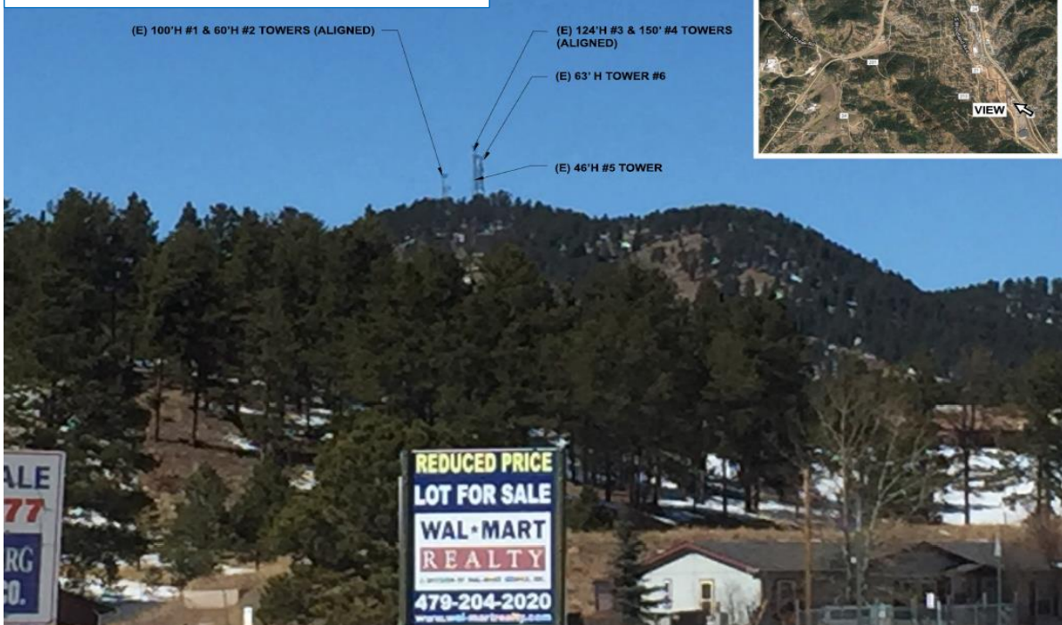
Figure 3c: Existing Site looking northwest
