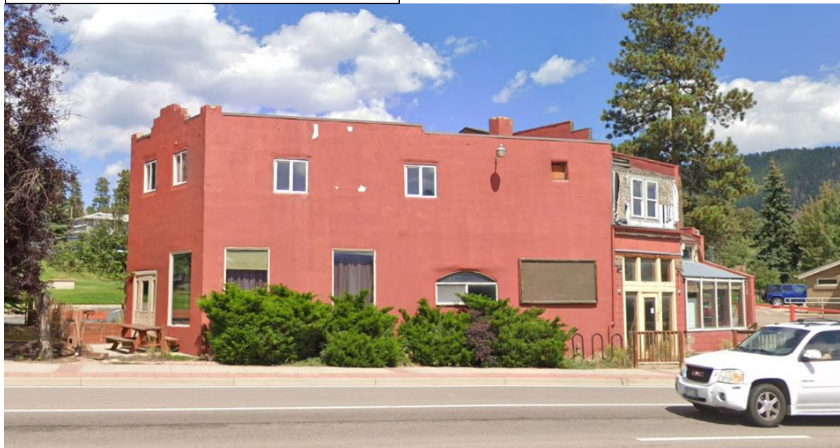
Figure 4: Vos Building 2024 – south elevation
