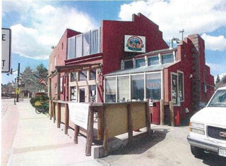
Figure 5-4: View of commercial building 5TL.4149. Looking west-northwest.
