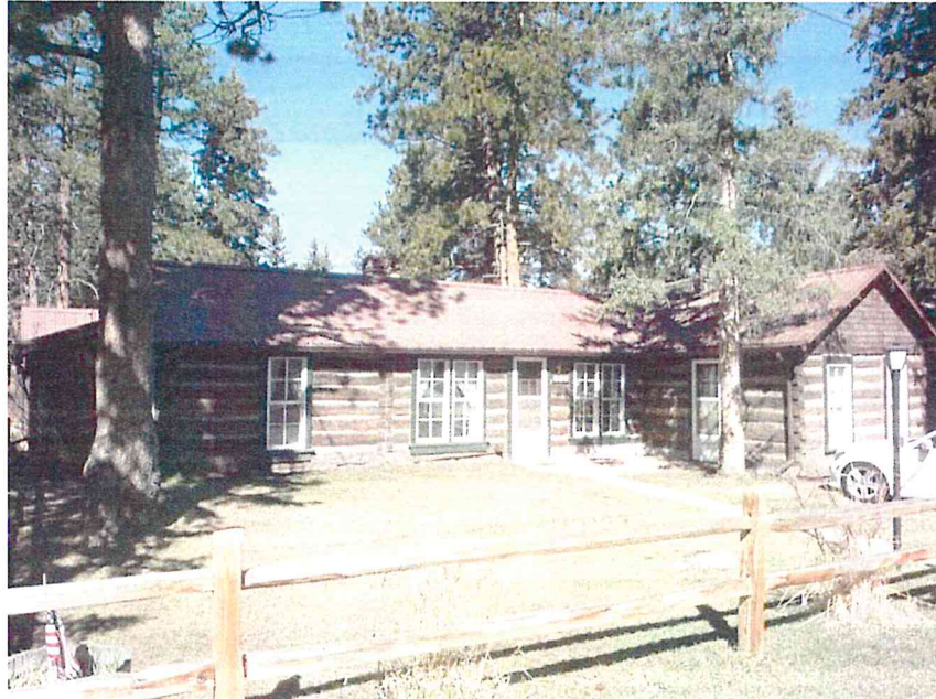
Figure 5-13: View of residence 5TL.4158. Looking west-northwest.
