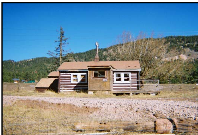
Junction House, 19600 N. Highway 24, 5TL3488, 1915.
