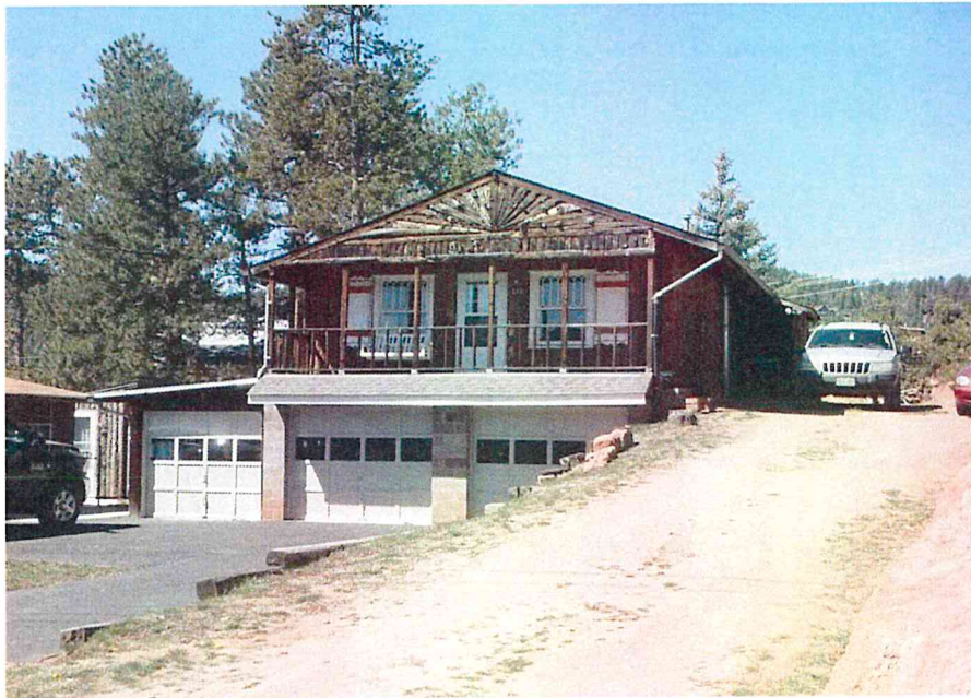
Figure 5-26: View of residence 5TL.4170. Looking west.
