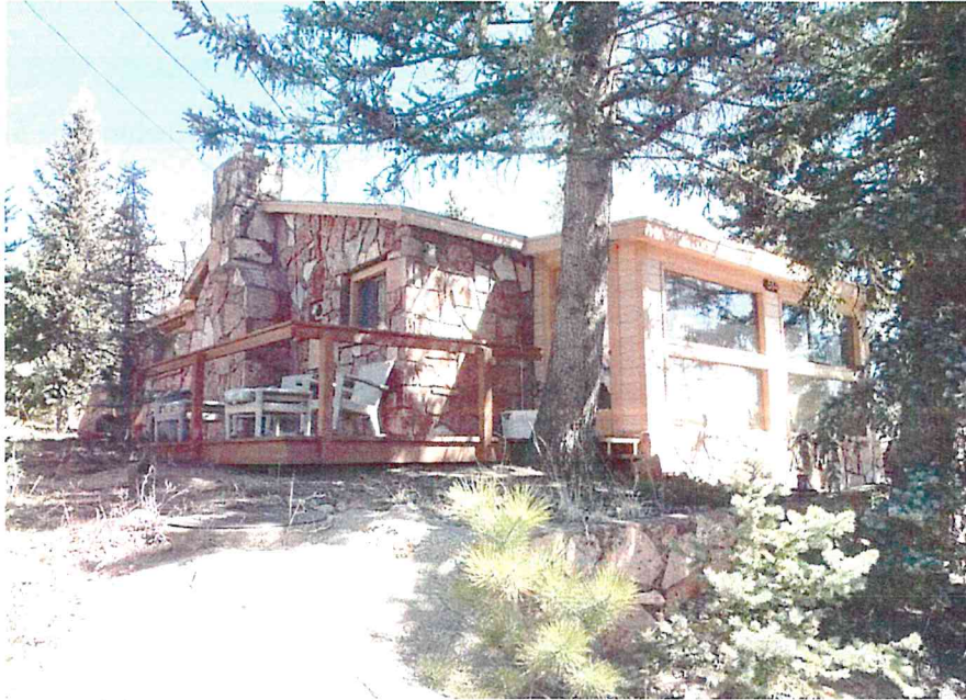
Figure 5-7: View of residence 5TL.4152. Looking northeast.
