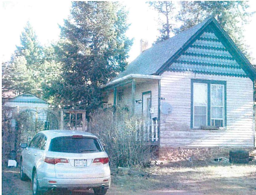
Figure 5-14: View of residence 5TL.4159. Looking north-northeast.
