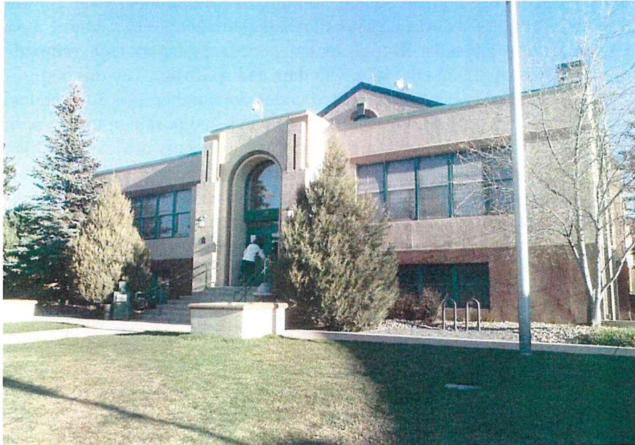
Figure 5-29: View of former middle school gymnasium 5TL.2529. Looking north.
