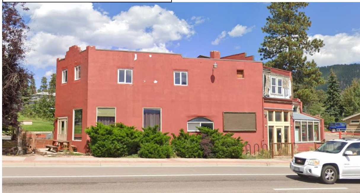
Figure 4: Vos Building 2024 – south elevation
