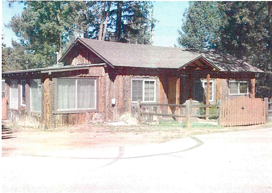
Figure 5-25: View of residence 5TL.4169. Looking northwest.
