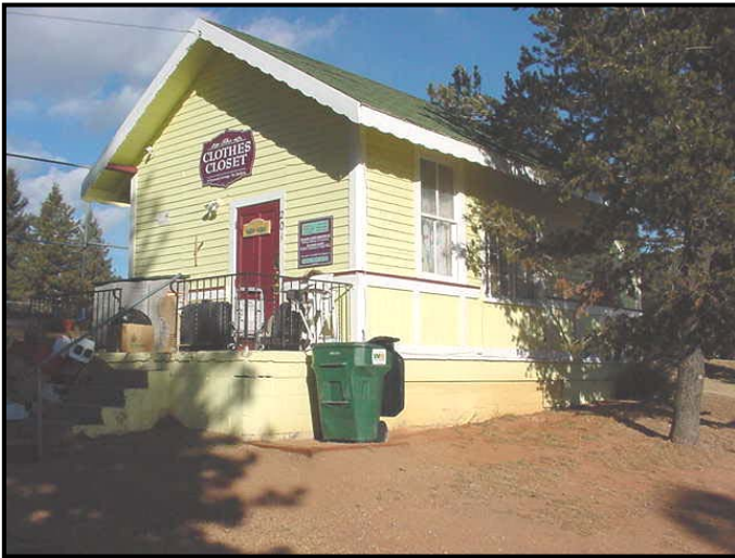
Midland Railroad Depot – Baggage, 201 Center Street, 5TL3466, 1903.
