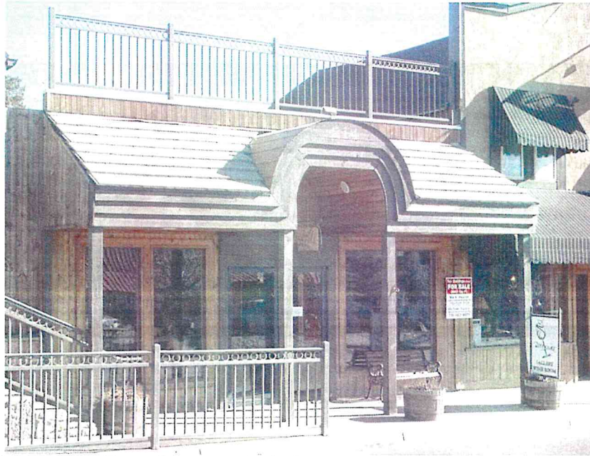
Figure 5-3: View of commercial building 5TL.4148. Looking northeast.
