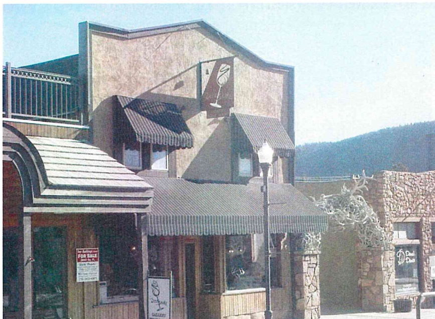
Figure 5-2: View of commercial building 5TL.4147. Looking northeast.
