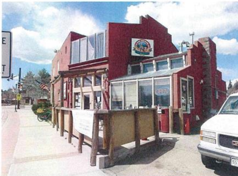
Figure 5-4: View of commercial building 5TL.4149. Looking west-northwest.
