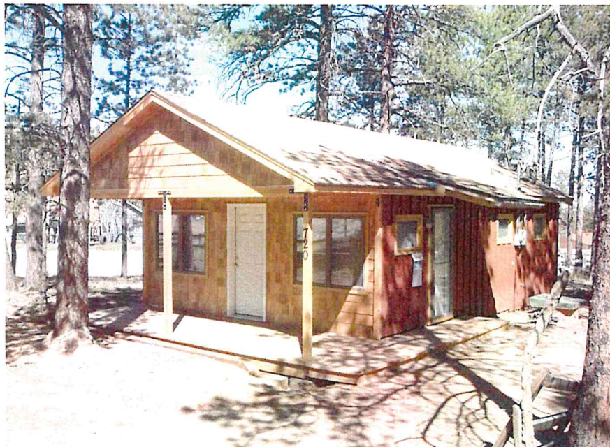
Figure 5-15: View of residence 5TL.4160. Looking northwest.
