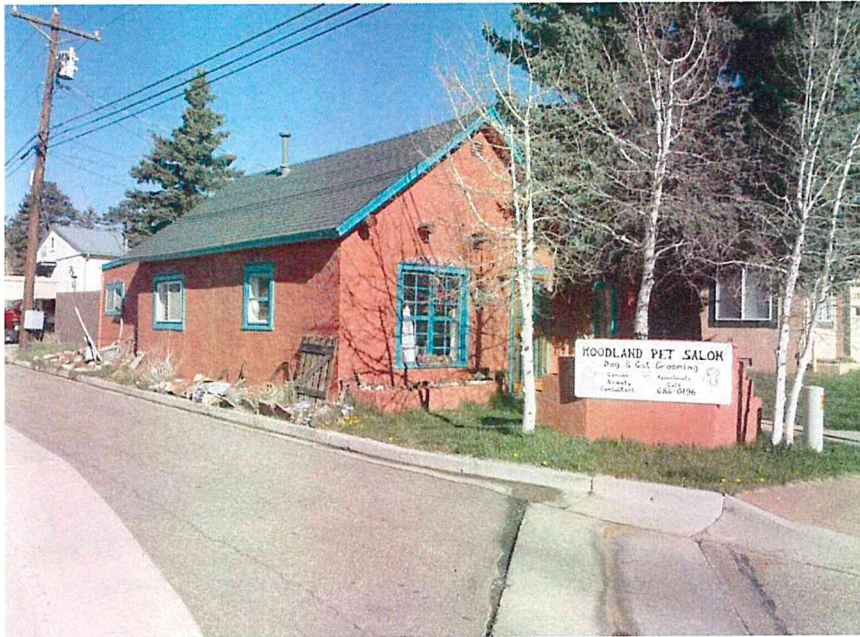
Figure 5-8: View of converted residence 5TL.4153. Looking northwest.
