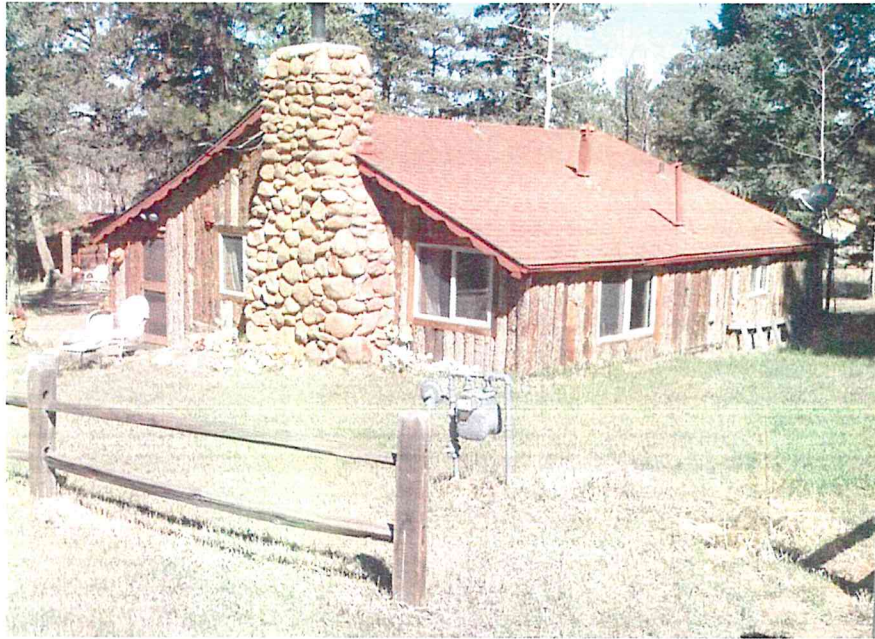
Figure 5-19: View of Residence 5TL.4163. Looking northwest.
