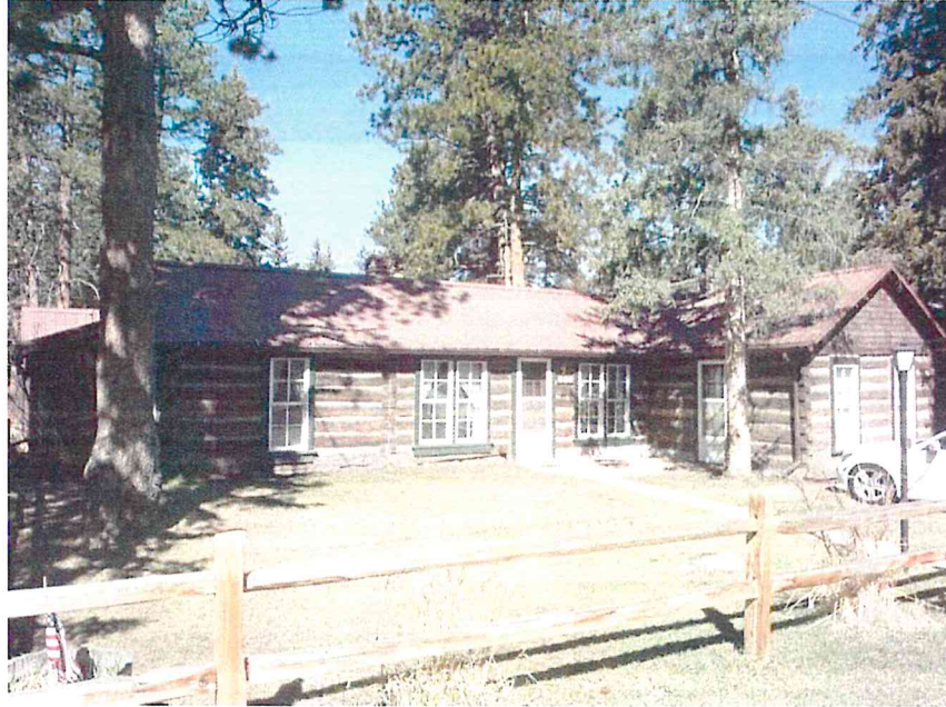
Figure 5-13: View of residence 5TL.4158. Looking west-northwest.
