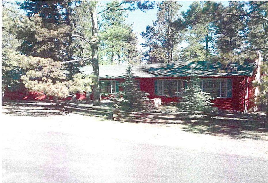
Figure 5-23: View of residence 5TL.4167. Looking northwest.
