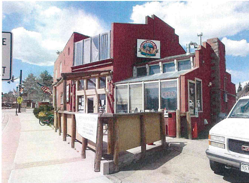
Figure 5-4: View of commercial building 5TL.4149. Looking west-northwest.
