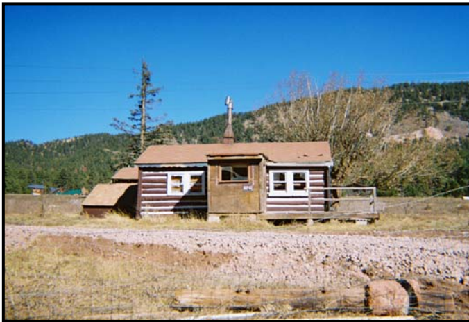
Junction House, 19600 N. Highway 24, 5TL3488, 1915.
