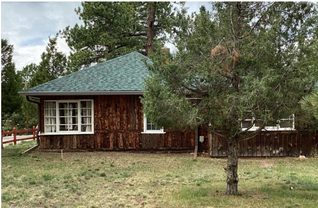
Figure 6: Griffith Cabin East Elevation 2026 – There is a large multi-lite casement window with sidelites on the east end of the gable addition and one 6/6 double hung window on the main house. There is a matching multi-lite casement window with sidelites at the east end of the porch.
