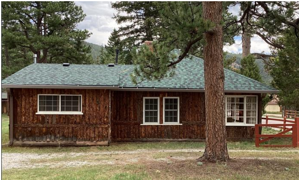
Figure 4: Griffith Cabin West Elevation 2026 – The porch wraps around on to this elevation at the south end and has another multi-lite casement window with sidelites. The main house has vertical log slab siding with a horizontal slab log siding band at about 3'-0" above grade. The windows on the oldest portion of the building is 6/6 double hung wood windows. The gable addition has a nine lite sliding window.
