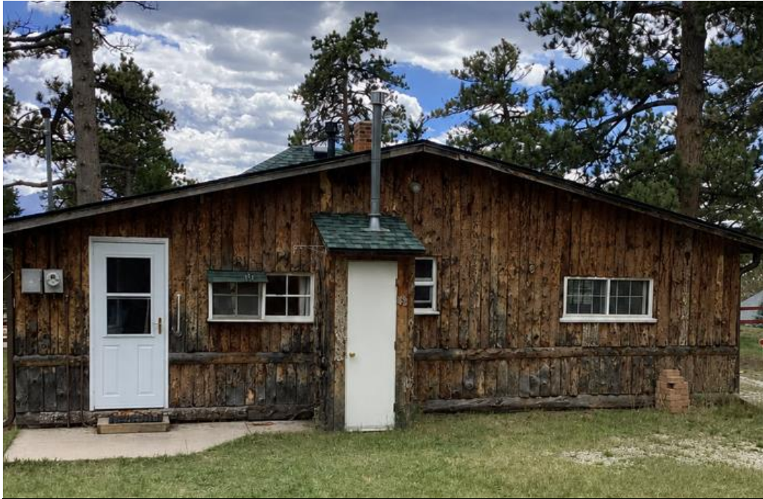
Figure 5: Griffith Cabin North Elevation 2026 – This is the gable end of the addition. There is a multi-lite entrance door into the kitchen, two small six lite slider windows and a small multi-lite window in the bathroom.
