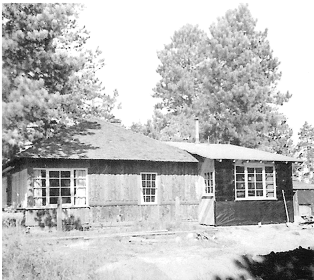
This 1949 photo shows the construction of an addition to the back of the house.
