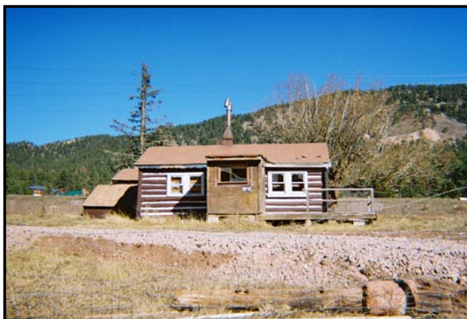
Junction House, 19600 N. Highway 24, 5TL3488, 1915.
