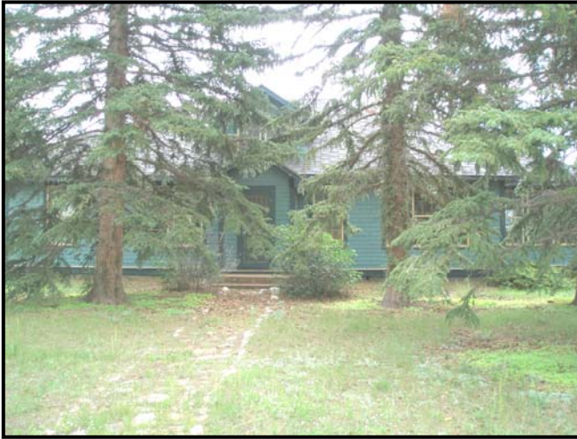
Bergstrom House, 110 E. Lake Street, 5TL.3469, 1925.
