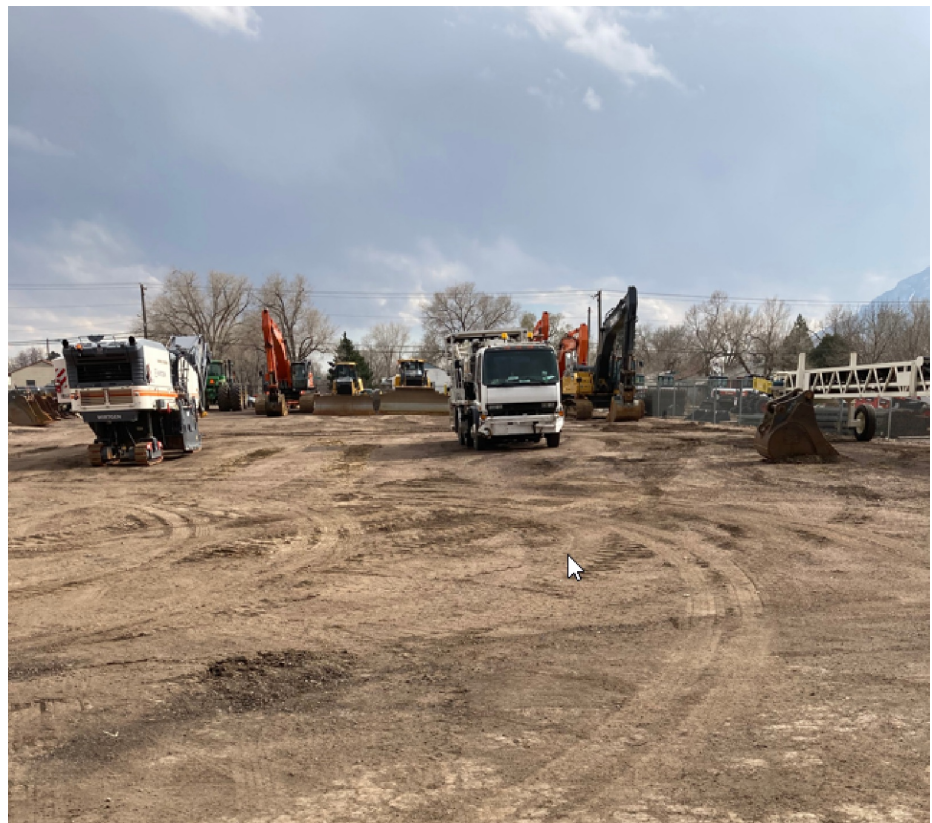
Heavy Equipment Yard
