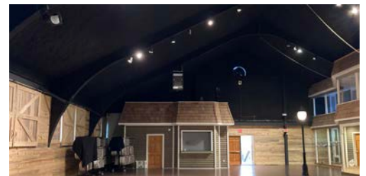
6 Ute Pass Cultural Center in need of facility upgrades.
