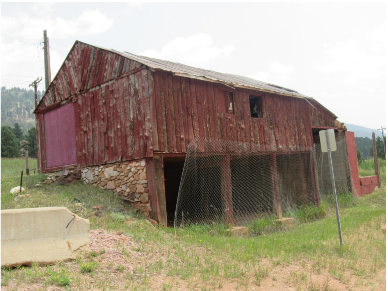
Northwesterly and Southwesterly Elevation of Barn
