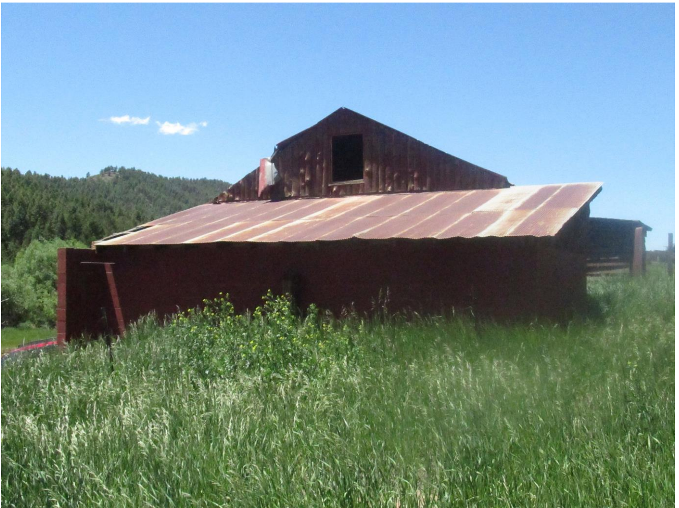
Northeasterly Elevation of Barn
